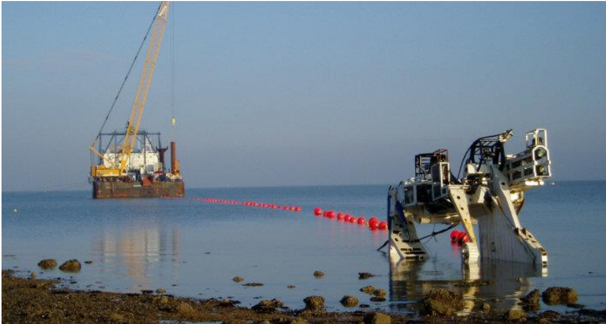
Figure 19: Global Marine's Hi-Plough
